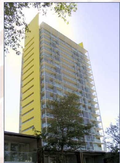
The Quarry, situated at Distillery Hill East (Site 1B), Pyrmont was completed in July 2004 and contains 95 units.
