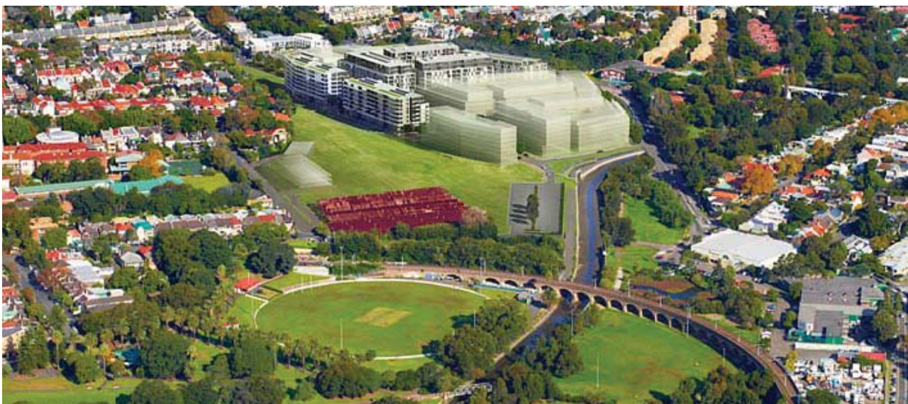
Figure 1.5 Harold Park development shown as a background to Johnstons Creek Parklands
