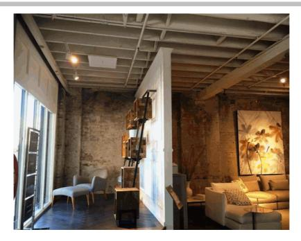
Caption: Interior of former warehouse showing original timber structure and exposed brick walls
