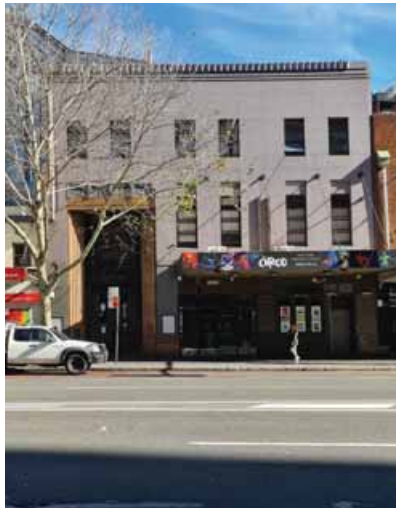
MIDBLOCK SITE 37-41 Oxford Street
