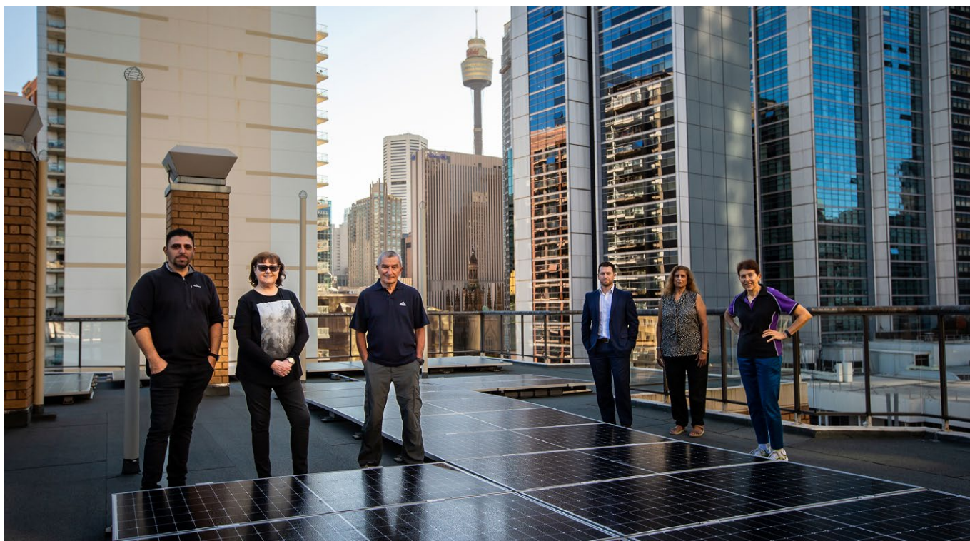
Smart Green Apartments partner Windsor Plaza and their rooftop solar array. Credit: Katherine Griffiths
