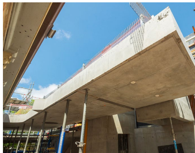
Pyrmont Community Centre under construction. Credit: Will Jones
