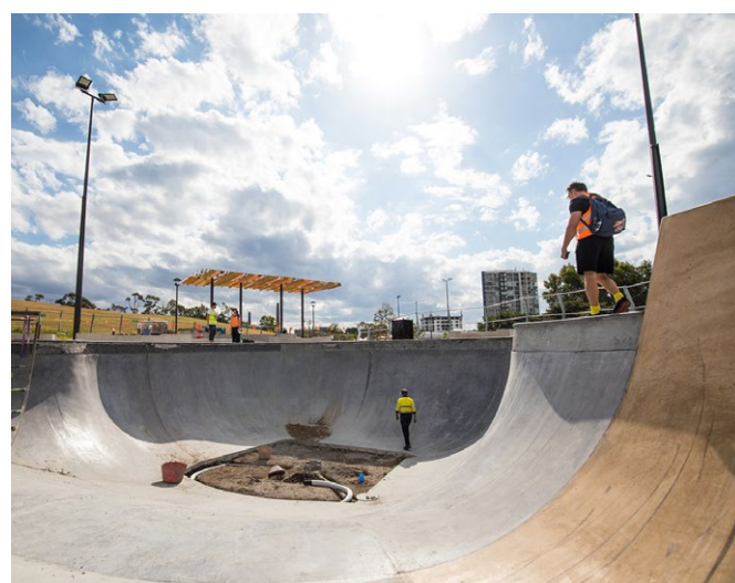
Skatepark bowl under construction, Sydney Park, Alexandria. Credit: Chris Southwood
