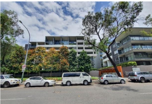
Figure 8 Powell Street facing South
