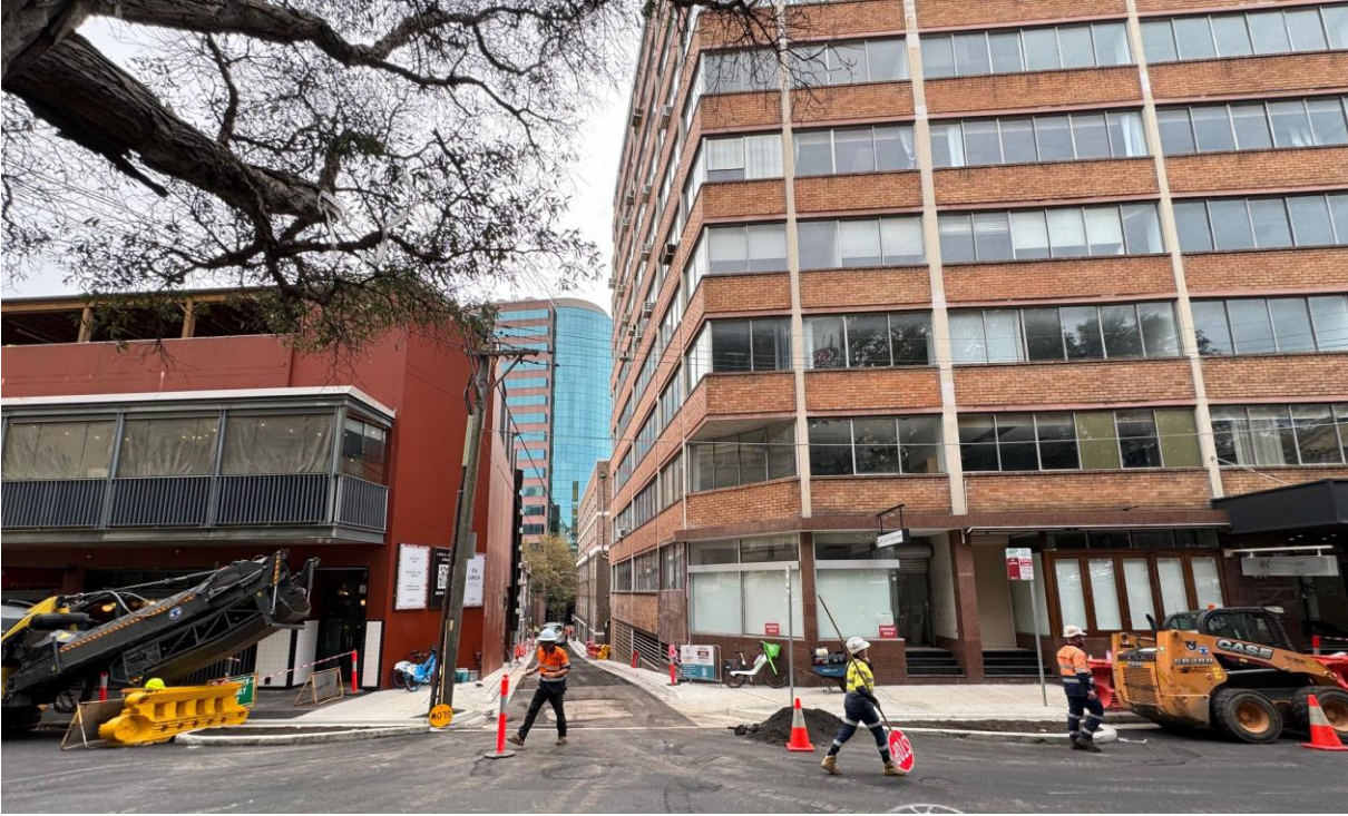
Figure 3. Looking towards the site as viewed along Terry Street
