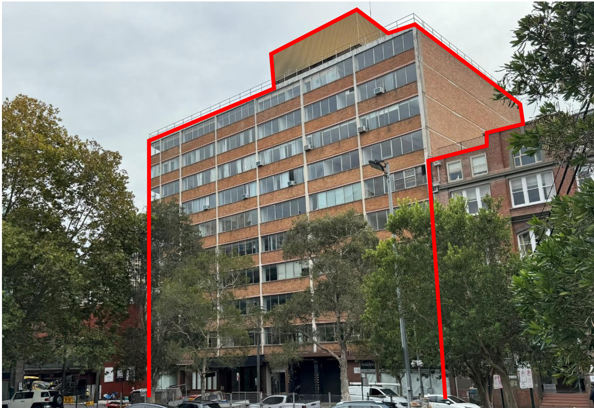
Figure 2: 8-24 Kippax Street, viewed from the south-east outlined in red
