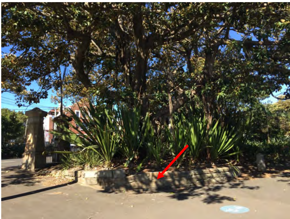
Plate 3.10 The western-most Moore Park Gateway piers (left) and the sandstone garden wall that will be retained (shown by red arrow) near the Korean War Memorial (view north-east)
