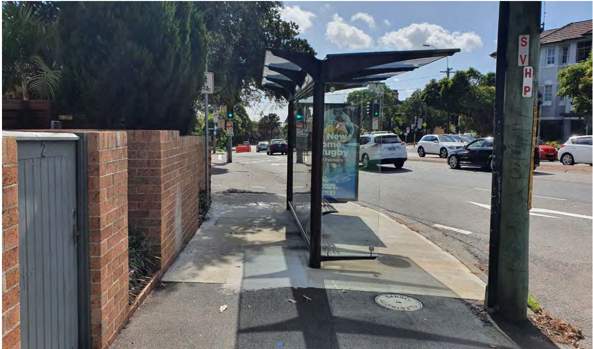
Photograph 6.1 Bus stop on Moore Park Road between Lang Road and Cook Road
