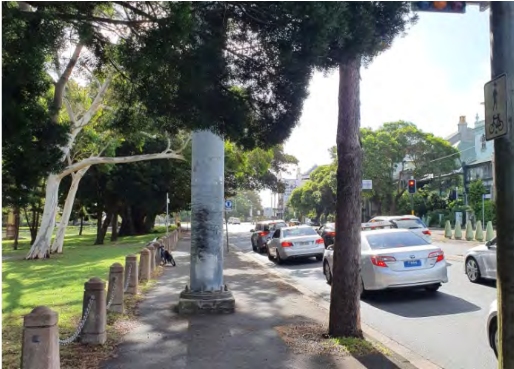
Photograph 6.5 Variable message sign base/footing within cycleway
