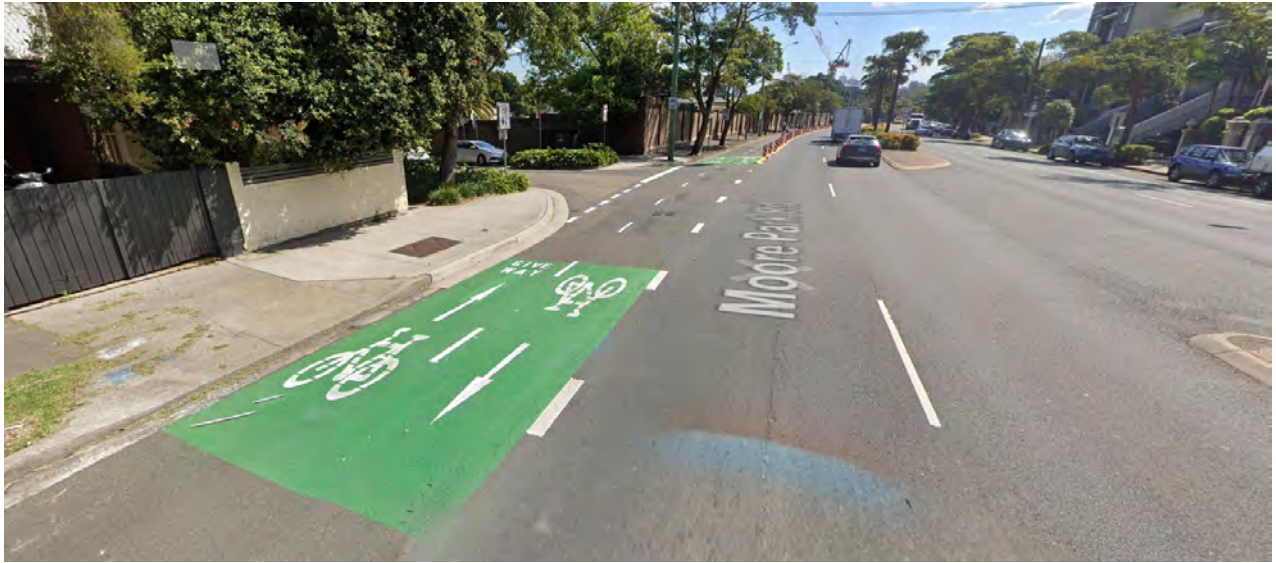
Photograph 6.2 Example of cycleway surface treatment
