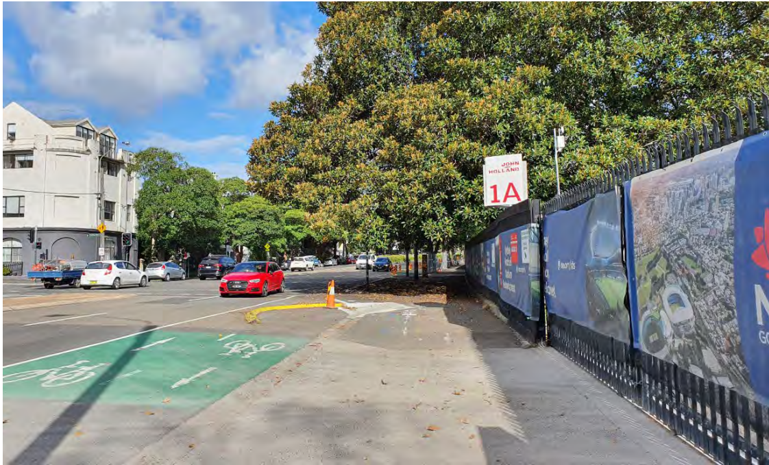
Photograph 6.4 Sydney Football Stadium construction access
