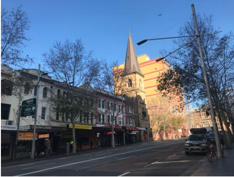
Figure 27: George Street opposite the site, looking south.
