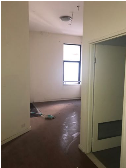
Figure 47: Nos. 761-763 George St First Floor interior.
