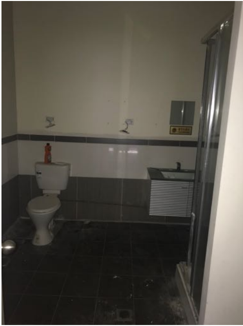
Figure 46: Nos. 761-763 George St First Floor interior.
