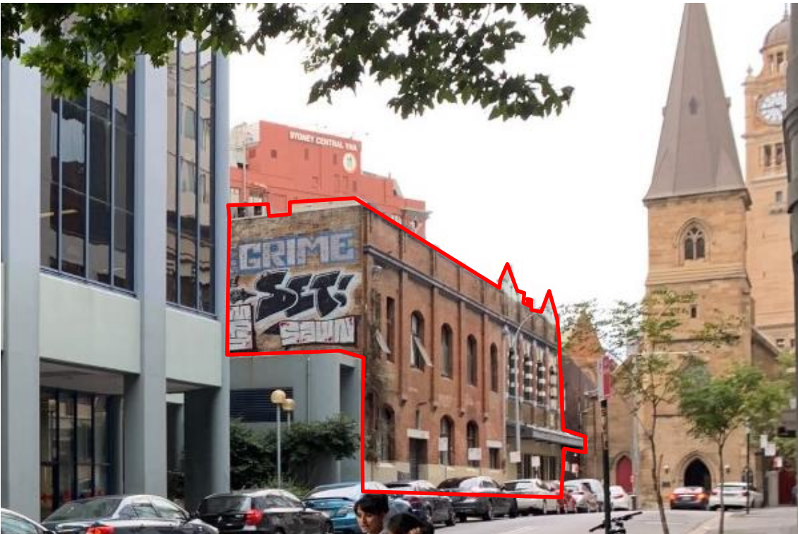
Figure 6. Looking east along Valentine Street towards subject site, shown in red
