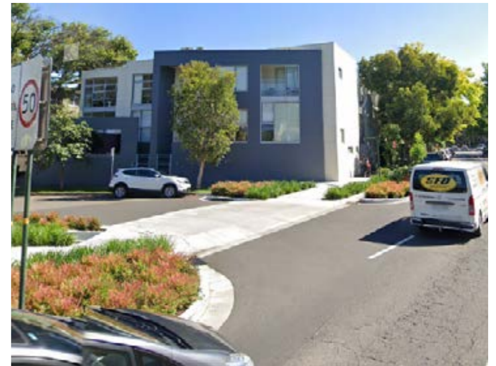
Example of continuous footpath treatment in Alexandria.
