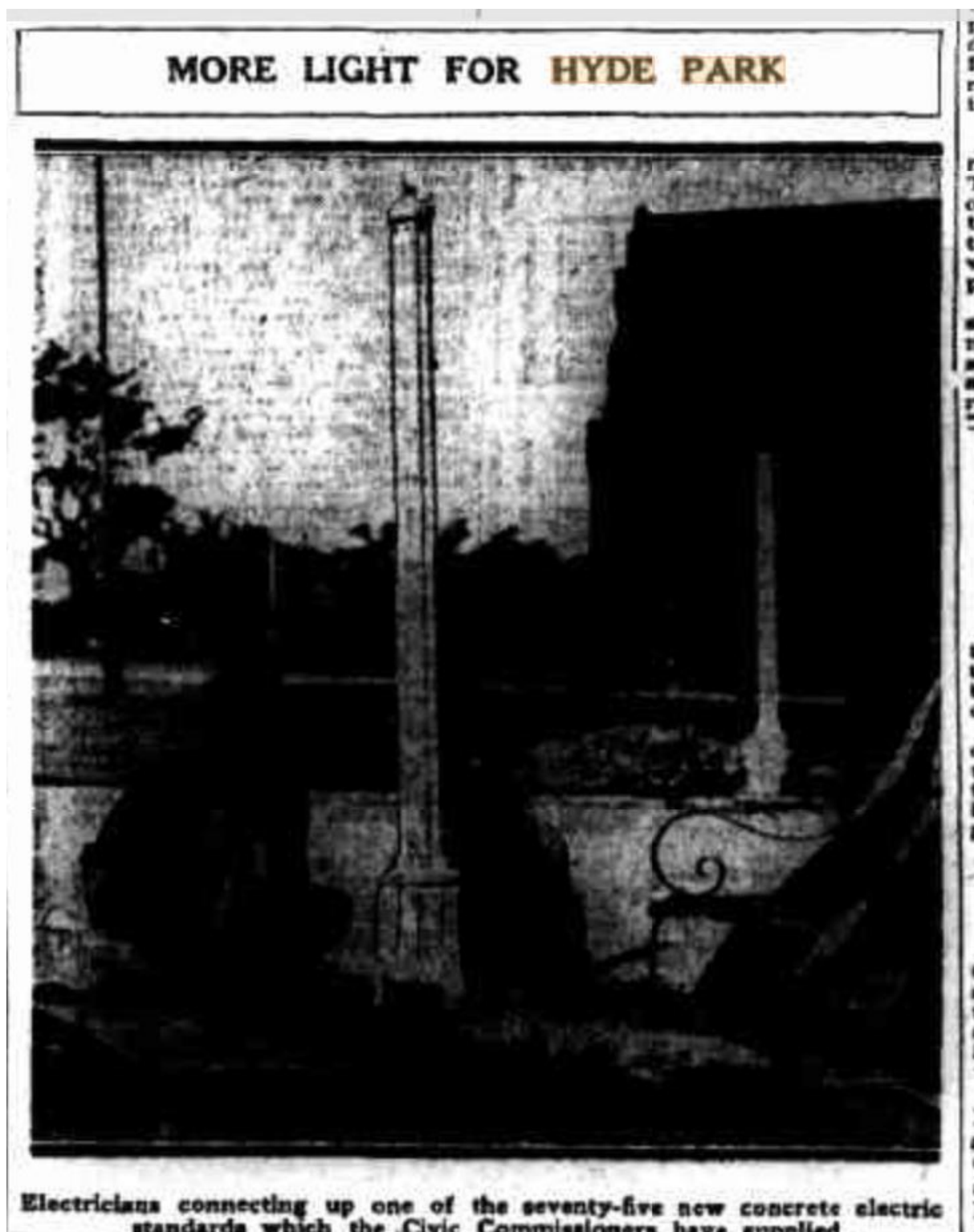
Figure 5.4 One of the concrete lighting standards being installed in Hyde Park. (Source: The Labour Daily 6 November 1929)
