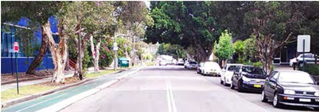
Figure 14 Bowden Street typical features (looking west near the proposed GS2AC)
