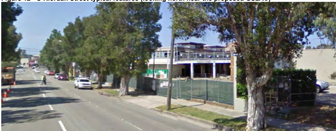
Figure 12 O’Riordan Street typical features (looking north near the proposed GS2AC)
