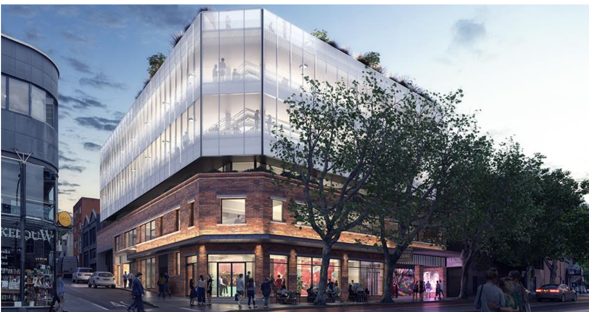
Figure 7. Alterations and vertical additions to 17 Oxford Street, Darlinghurst for office, cultural and creative uses.
