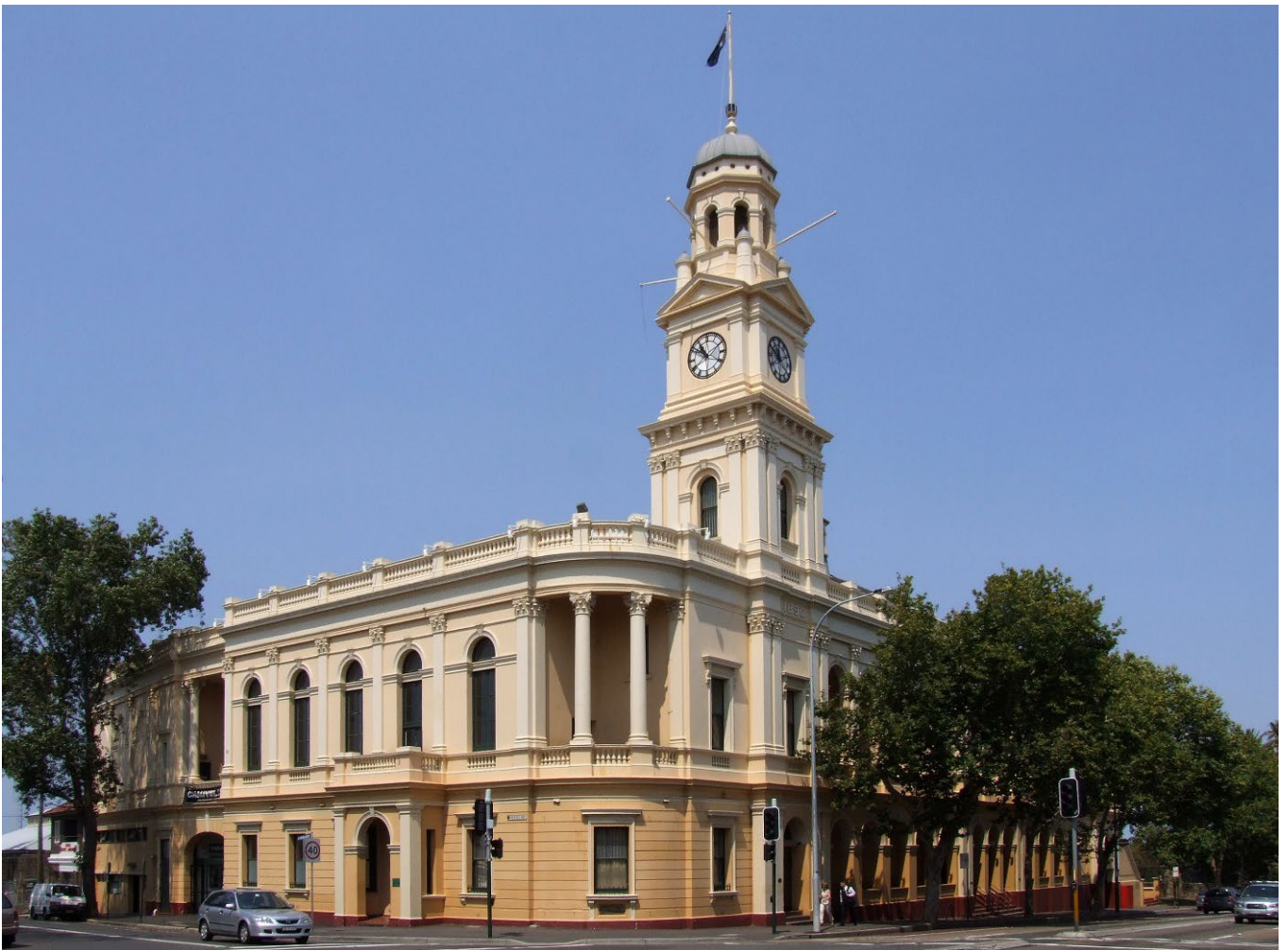
Figure 1. Paddington Town Hall – Photo by Paul Patterson / City of Sydney Fees and Charges Appendix 1 – 2
