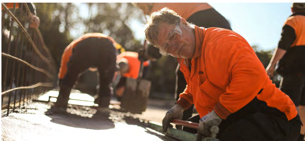
Image: Council staff renewing a footway
