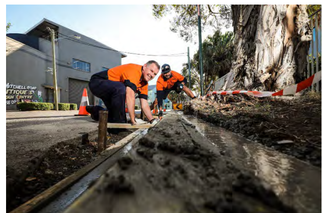
Image 26: Infrastructure Maintenance, Alexandria
