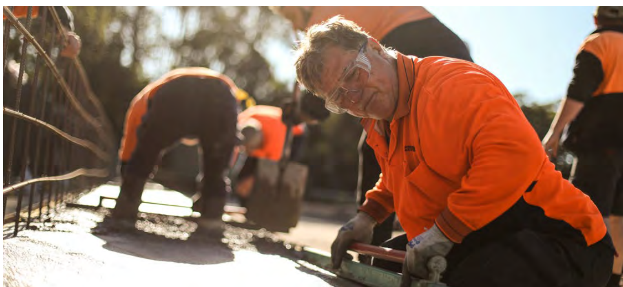
Image: Council staff renewing a Footpath
