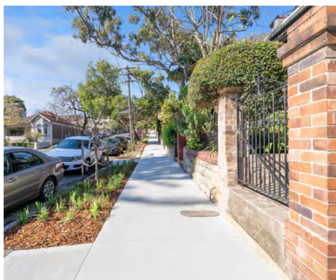
Images: Eglinton Road, Glebe Footpath Renewal Works 2021
