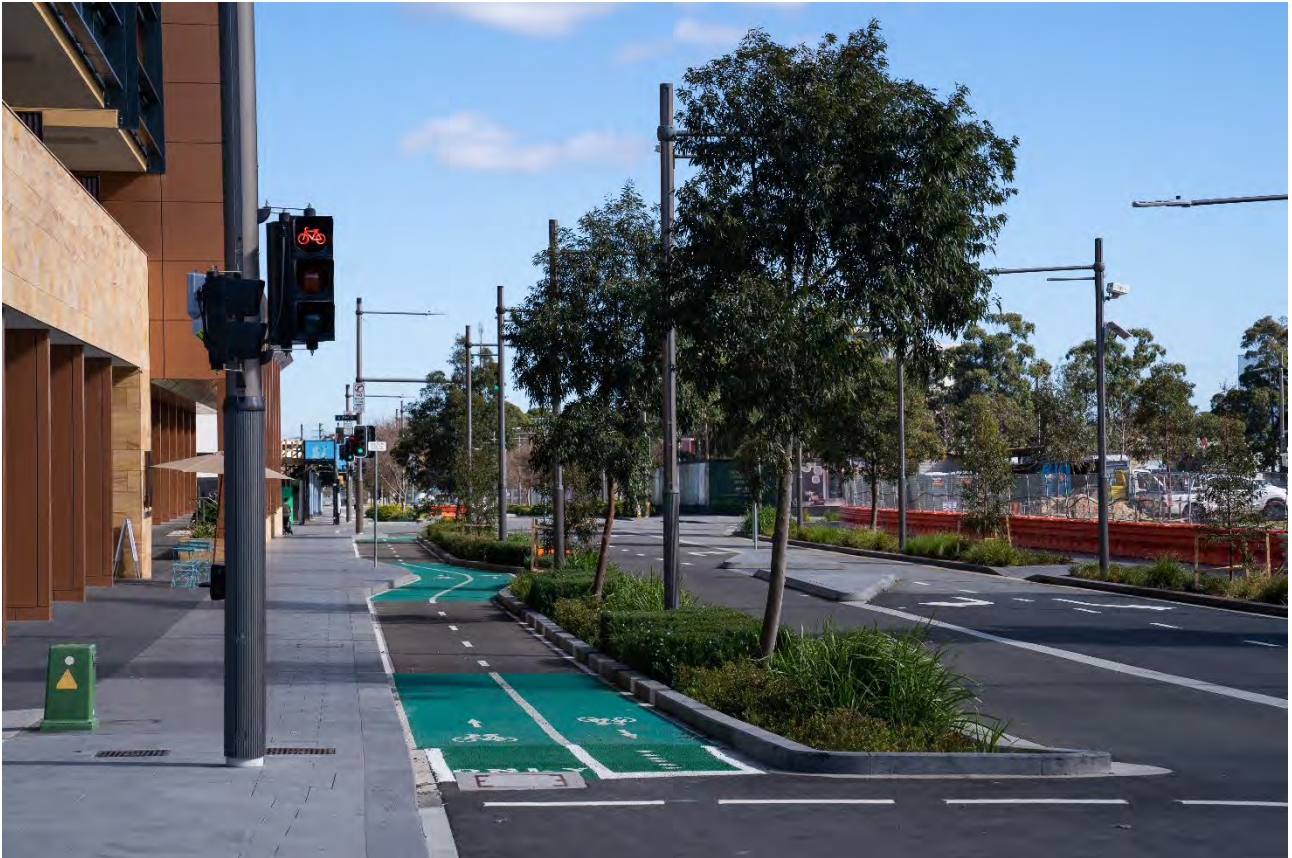
The Green Square trunk drain runs under Geddes Avenue, reducing flood risk in the area (Photo by Abril Felman / City of Sydney)
