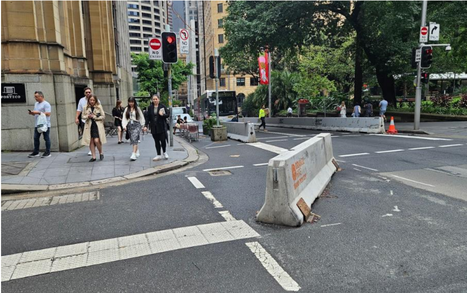
Example of temporary traffic calming at intersections prior to ultimate arrangements being delivered – York Street / Margaret Street Sydney CBD
