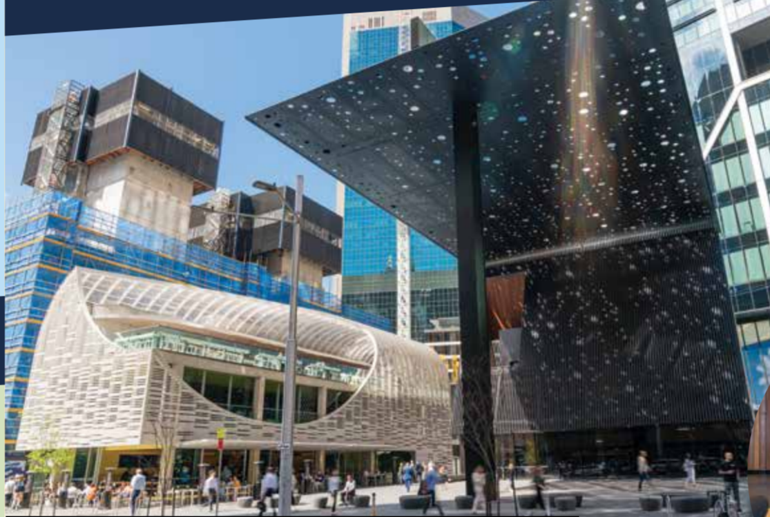
180 George Street Daniel Boyd artwork and Sir David Adjaye community and cultural building
